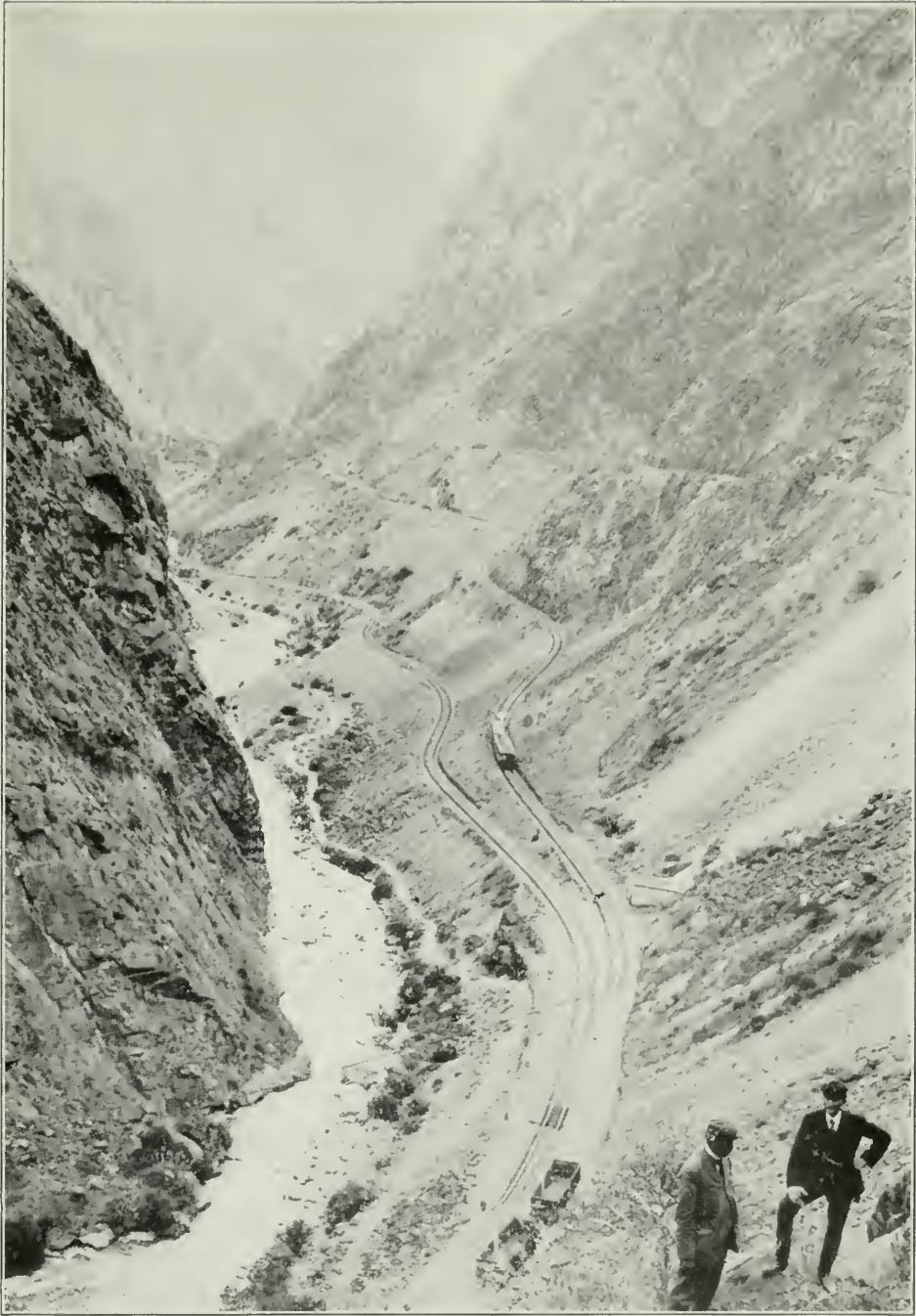
AMONG THE MOUNTAINS ON THE PERU CENTRAL RAILWAY. NOTE THE SWITCHBACKS AND ZIGZAG STYLE OF TRACK.
